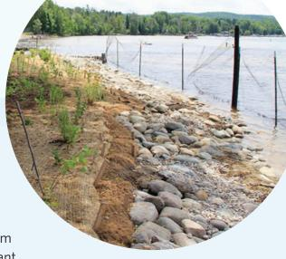
It can be used to restore a shoreline where native vegetation has been removed. Bioengineering provides fish and wildlife habitat and water quality benefits that may be lost with other stabilization methods. It can be designed in conjunction with riprap for high energy systems, allowing the shoreline to be stabilized while providing additional benefits to the lake ecosystem.
